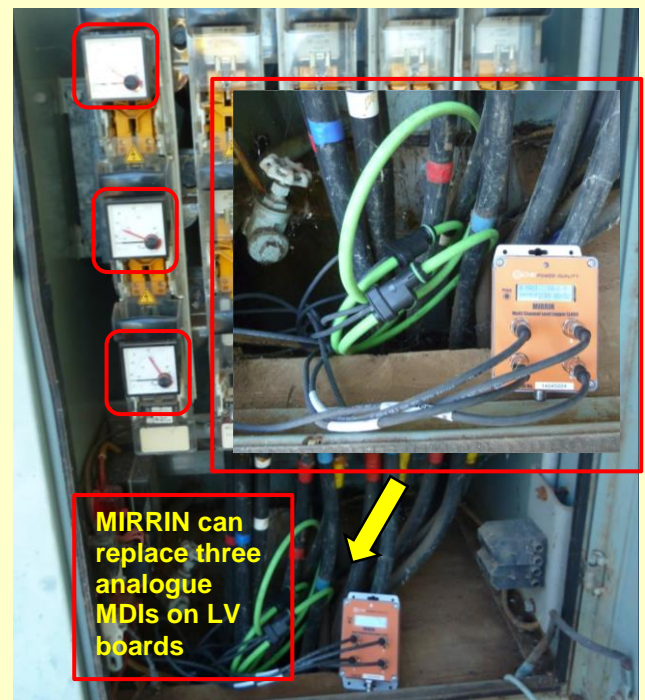
Figure 2: Installation - kiosk transformer
