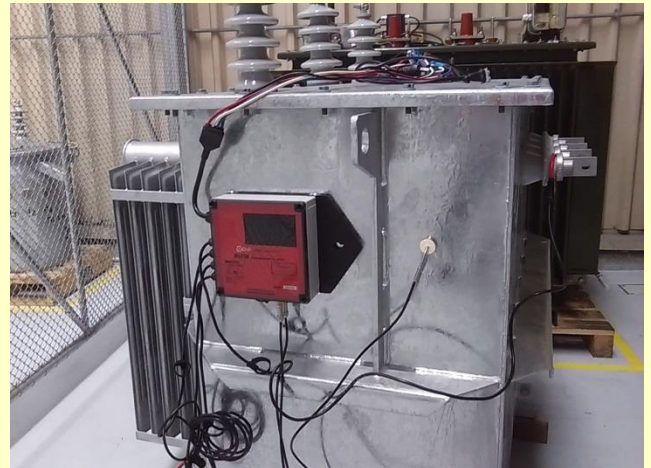
Figure 2: MATTINA - Installed on a distribution transformer
